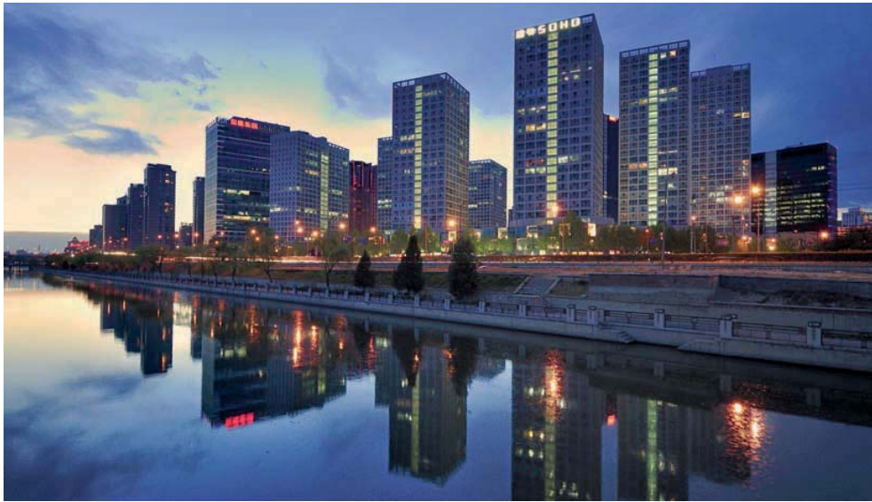
Real estate offers good, but not absolute protection against inflation (office building in Beijing).
